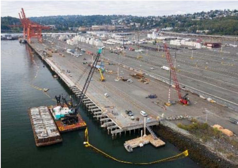
Dock Demolition Underway
