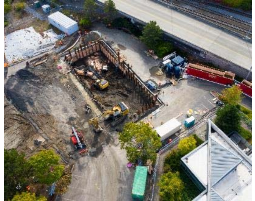
Primary Substation Excavation
